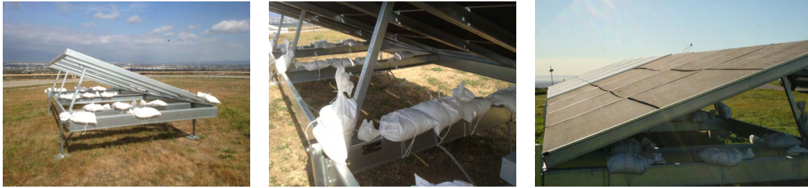
Photo 10: Sand Bags Tied to Unit 1 and Unit 2 to Simulate Actual Weight of Solar Unit
