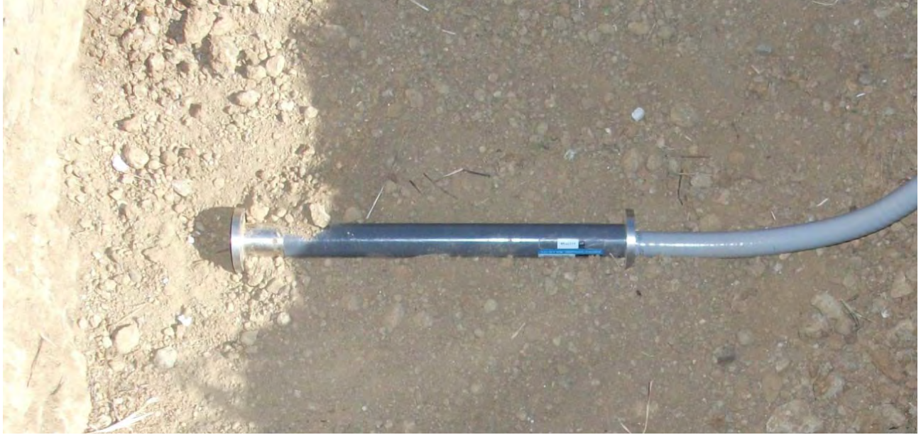
Photo 4: Geokon Deformation Sensor Placed Inside a Trench
