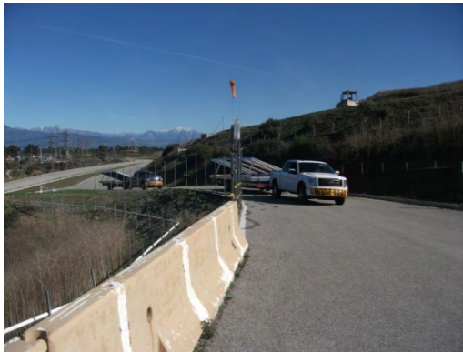
Units 1 and 2 arriving at the Site
